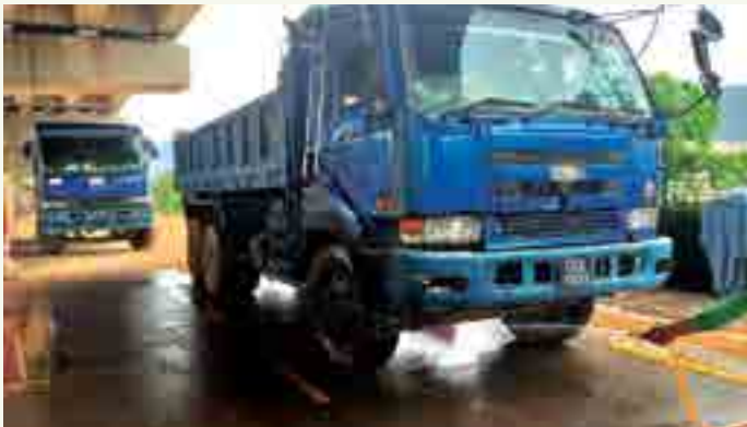
Tyre cleaning at the entrance before entering public road
