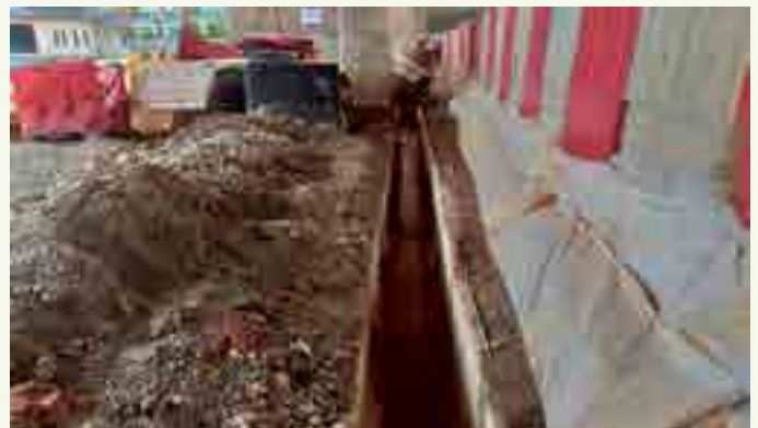
Maintenance of Project Hoarding
